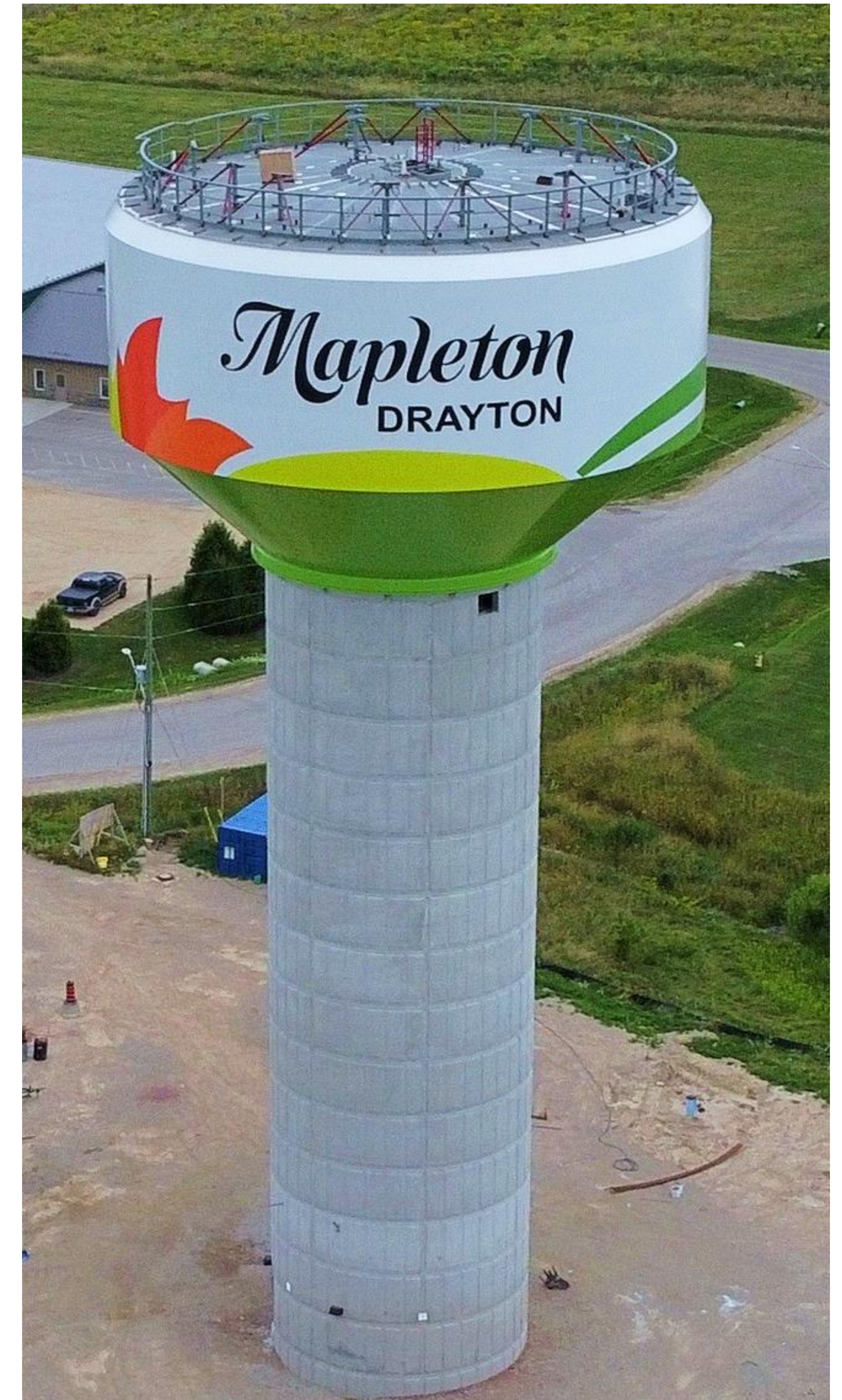
Drayton Elevated Tank
