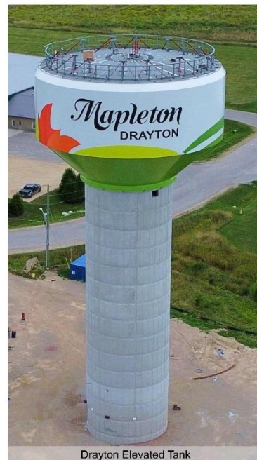
Drayton Elevated Tank
