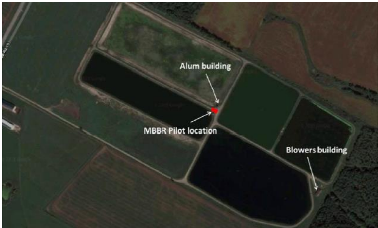
Figure 8-1: Location of MBBR Pilot Unit
