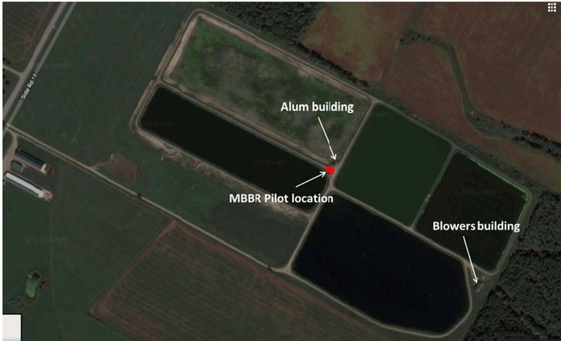
Figure 3-1 Location of the MBBR pilot unit
