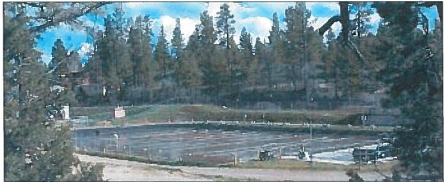
A single basin Biolac Wave Oxidation system in Arizona.
