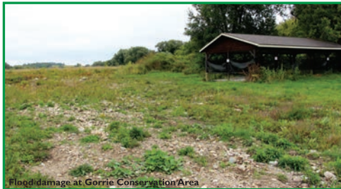
Flood damage at Gorrie Conservation Area
