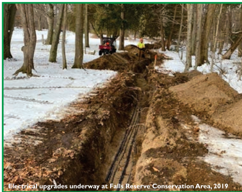
Electrical upgrades underway at Falls Reserve Conservation Area, 2019
