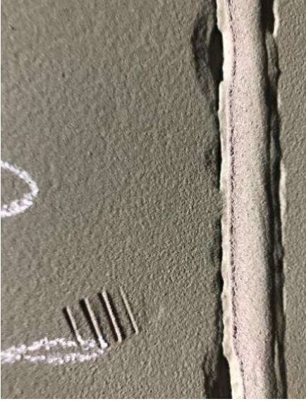
Weld Defect – Repairs Required
