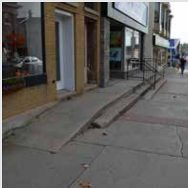
Ramps without handrails provide obvious challenges.
