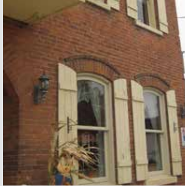
Wood shutters with curved top and decorative finishes.
