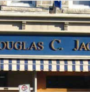
Extruded letters painted gold. Note retracted awning.
