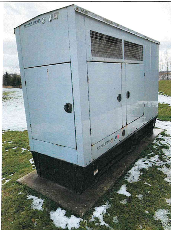
Phot PE7: Genset. Fair Condition, Does Not Meet TSSA Code.
