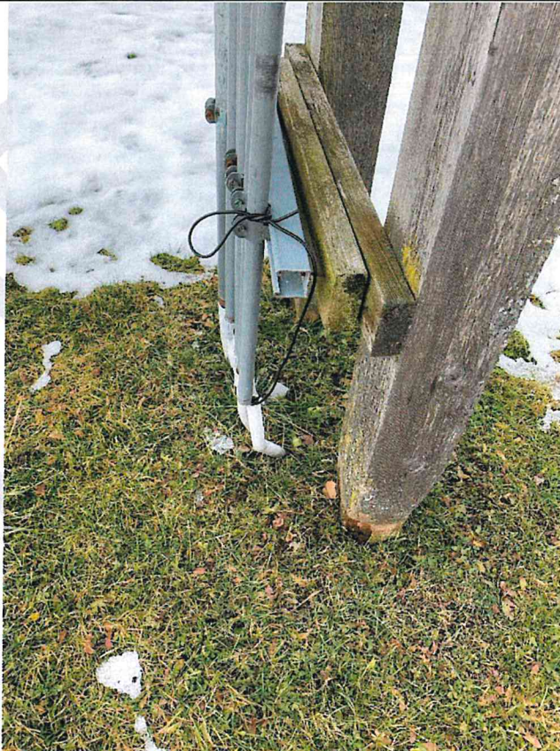
Photo BE8: Building Conduits (Exterior). Conduits Broken/Misaligned Entering Panel and Wells.
