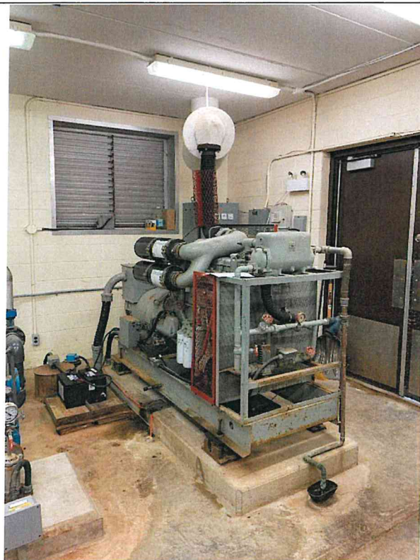
Photo PE1: Genset. Poor Condition, Consider Immediate Replacement.
