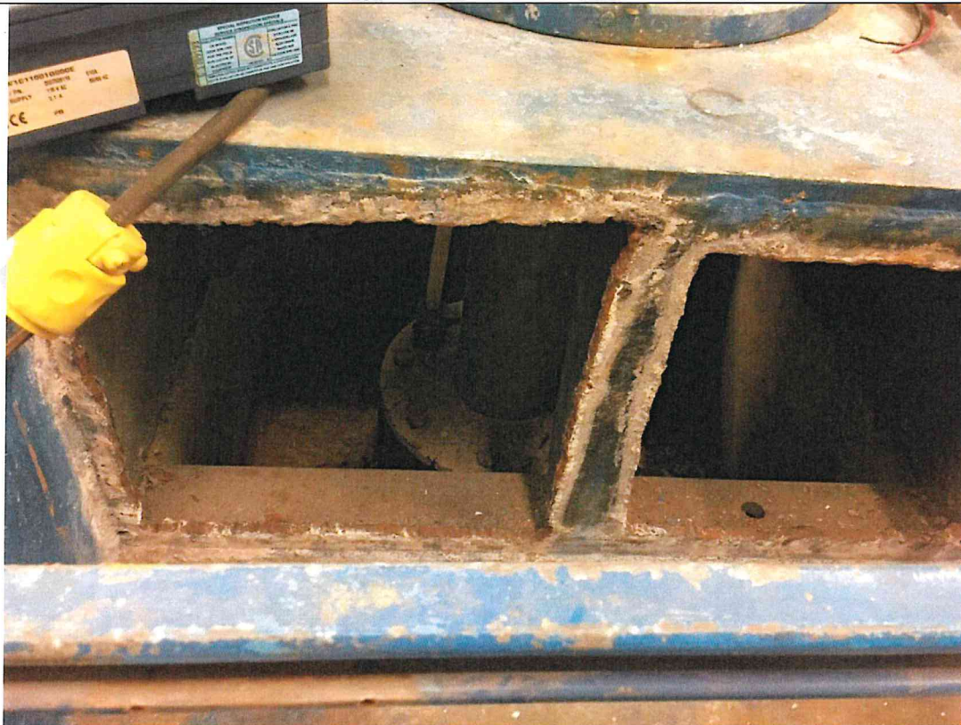
Photo PPE1: Well 1 Pump. Based in Heavily Corroded.
