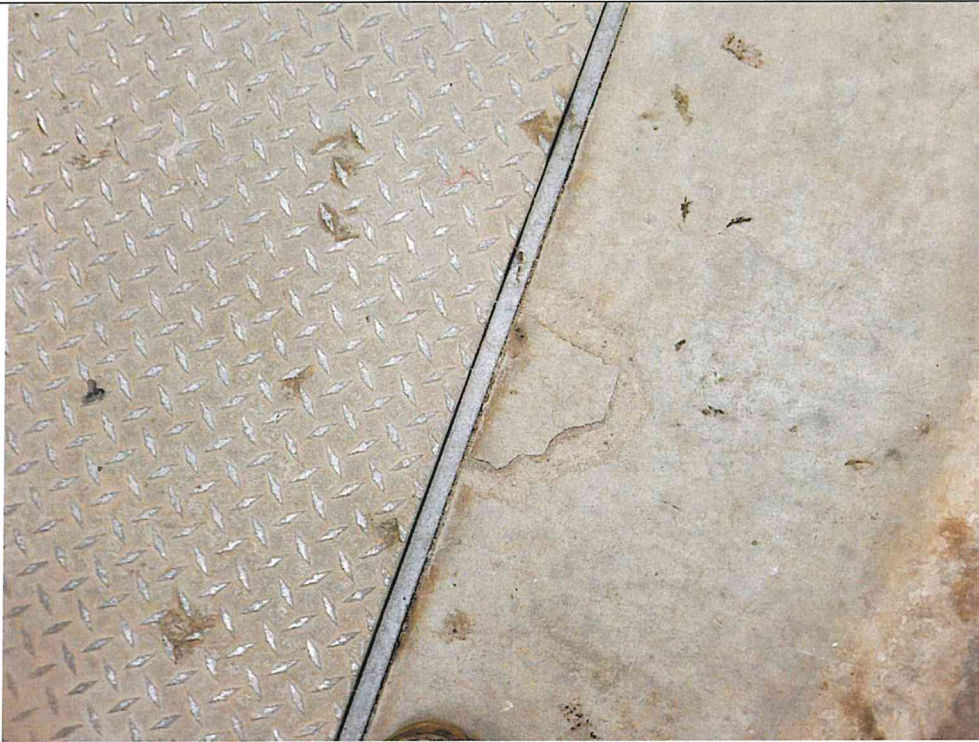
Photo S3: Reservoir Suspended Slab inside Pumphouse. Minor Spalls
