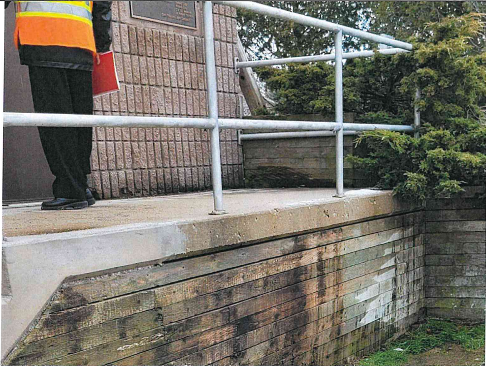
Photo S17: Exterior Aluminum Guardrail. Surface Rust on Wall Anchors
