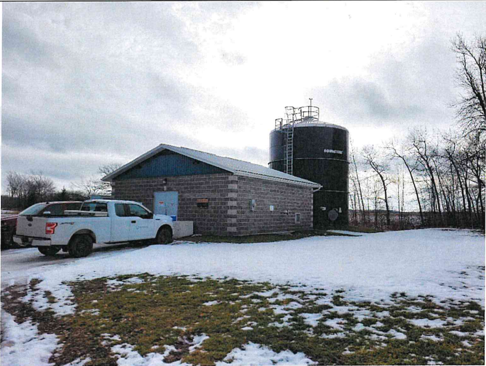
Photo S28: Moorefield Pumphouse
