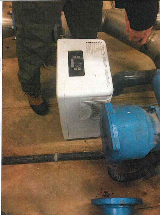
Photo M2: Portable Dehumidifier. Good Condition, but Lacks Capacity to Dehumidify Entire Space.
