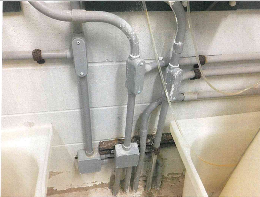
Photo BE7: Building Conduits (Interior). Conduit Mounts in Chemical Room Heavily Corroded.
