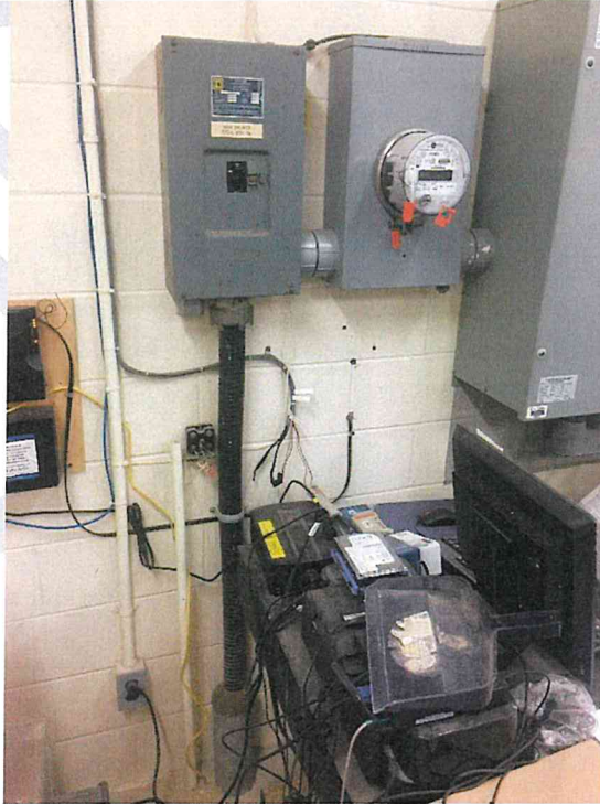
Photo BE4: Main Circuit Breaker. Rusting Observed on Breaker Enclosure. Improper Storage of Desk within Unsafe Proximity of Electrical Equipment.
