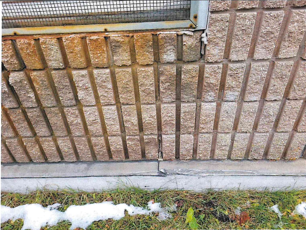
Photo S24: Block Veneer. Spalled Mortar.
