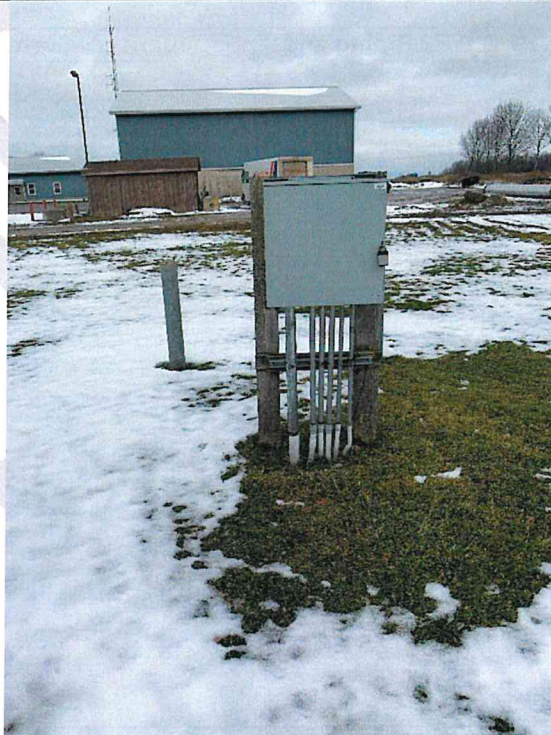
Photo PE8: Well Control Panel. Panel and Mounting Structure in Poor Condition.
