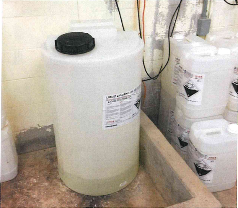
Photo PPE14: Sodium Hypochlorite Pumps and Storage Tanks. Area and Tank are Not Properly Ventilated. Health and Safety Issues for Delivery.
