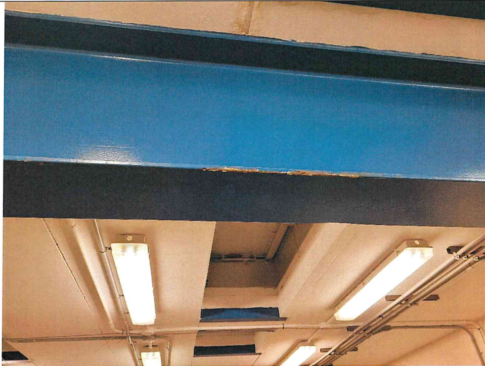
Photo S15: Roof Steel Beam. Surface Rust & Chipped Coating
