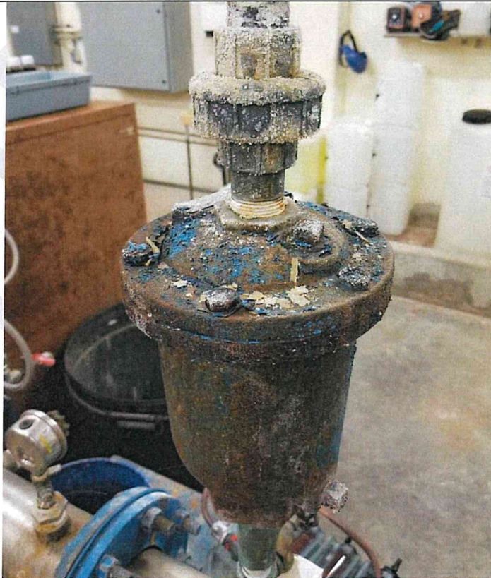
Photo PPE3: Well 2 Air Release Valve. Heavily Corroded.
