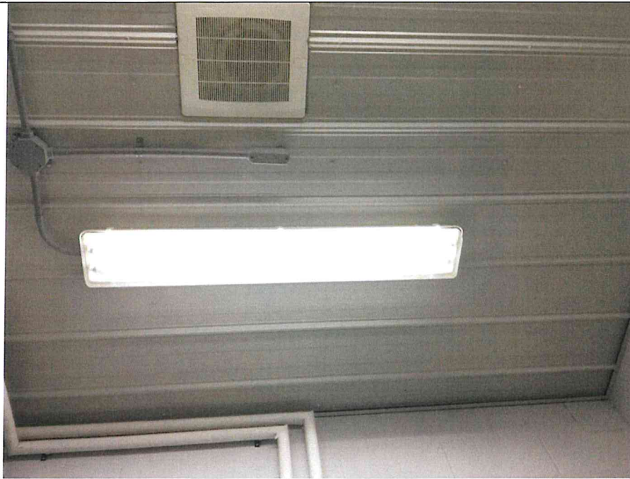
Photo M5: Exhaust Fan (Chemical Room). Functioning, but Relies on Hand-Written Note on Door to Prevent Being Shut Off; Lacks Effective Capacity.
