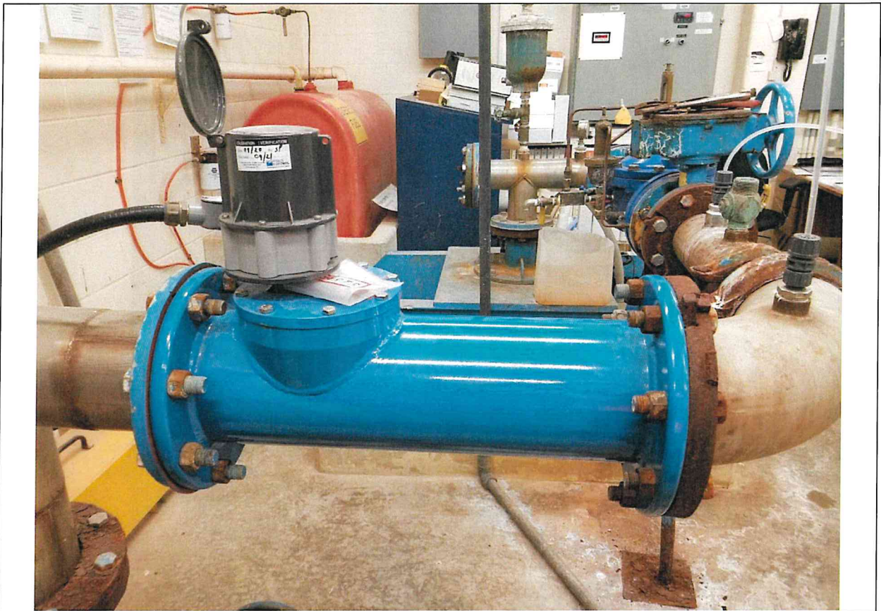
Photo PI6: Flowmeter for Well Pump 1. Old Cable-Style Flowmeter.
