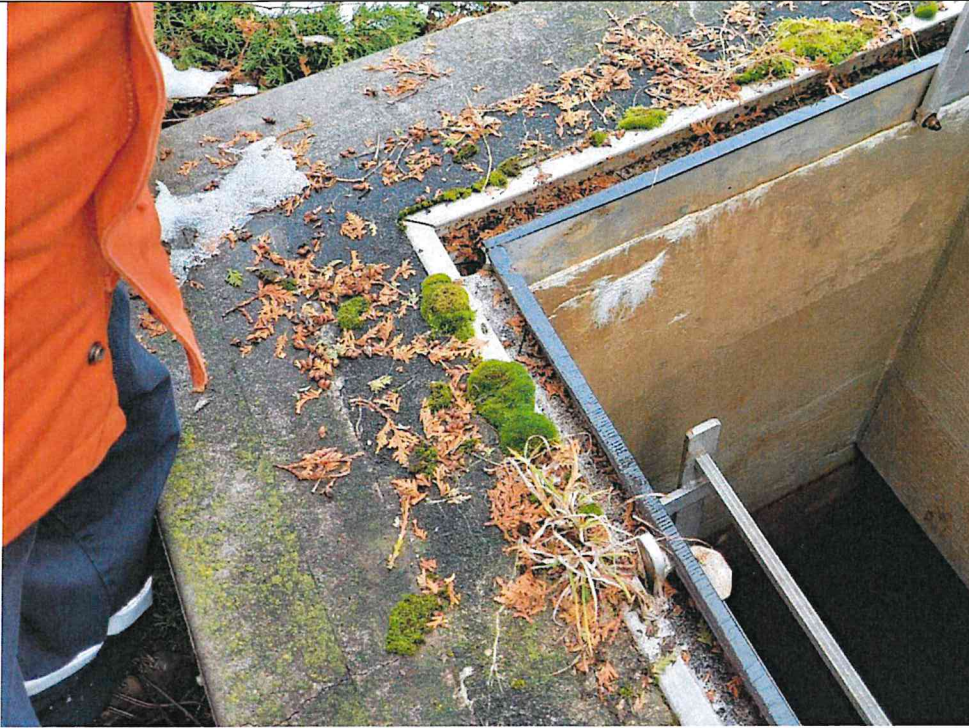
Photo S7: Reservoir Access Hatch. The Operator Reported the Hatch Drain to be Clogged
