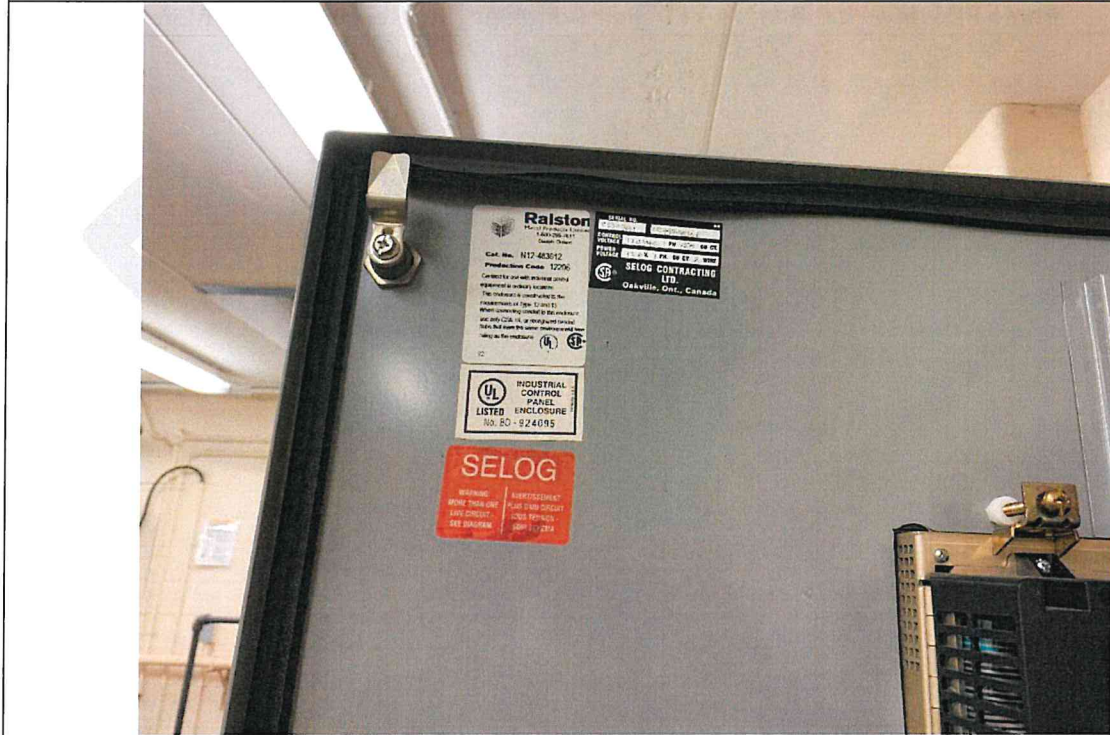
Photo PE6: PLC Control Panel. Door Weatherstripping Faulty. Consider Replacing Immediately Given High Humidity Within Room to Extend Life of PLC.
