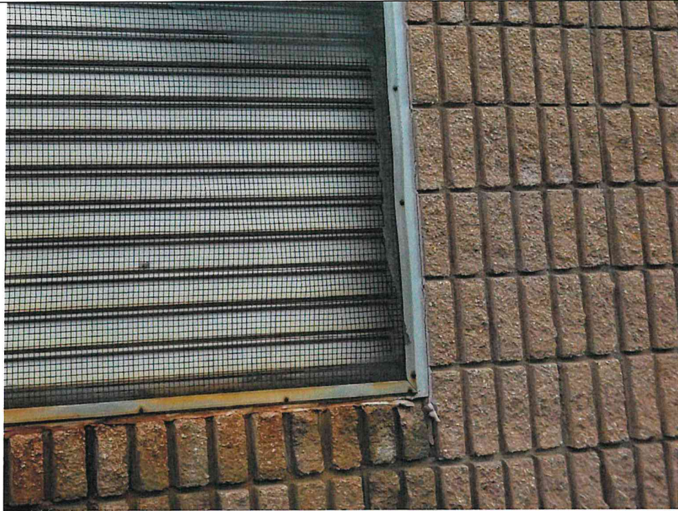
Photo S27: Metal Louvers. Sealants Around Louver Have Failed.
