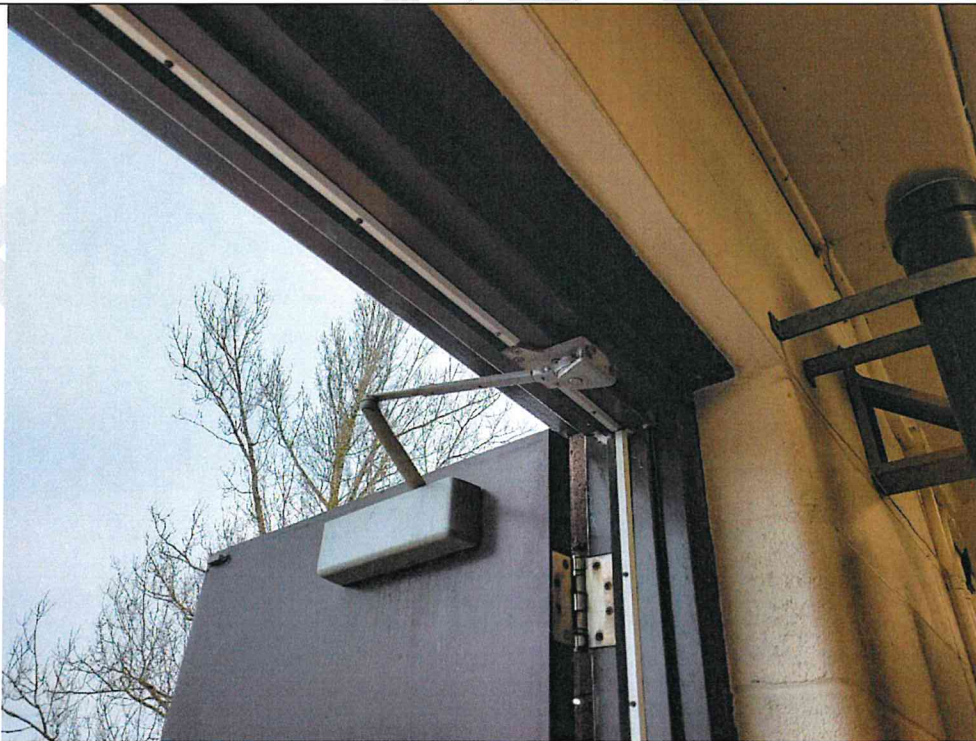
Photo S26: Exterior Metal Double Door. Hardware has Minor Rusting
