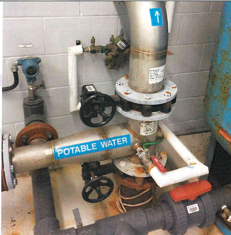
Photo PPE27: Isolation Discharge Valve and Blowoff. Heavy Corrosion.
