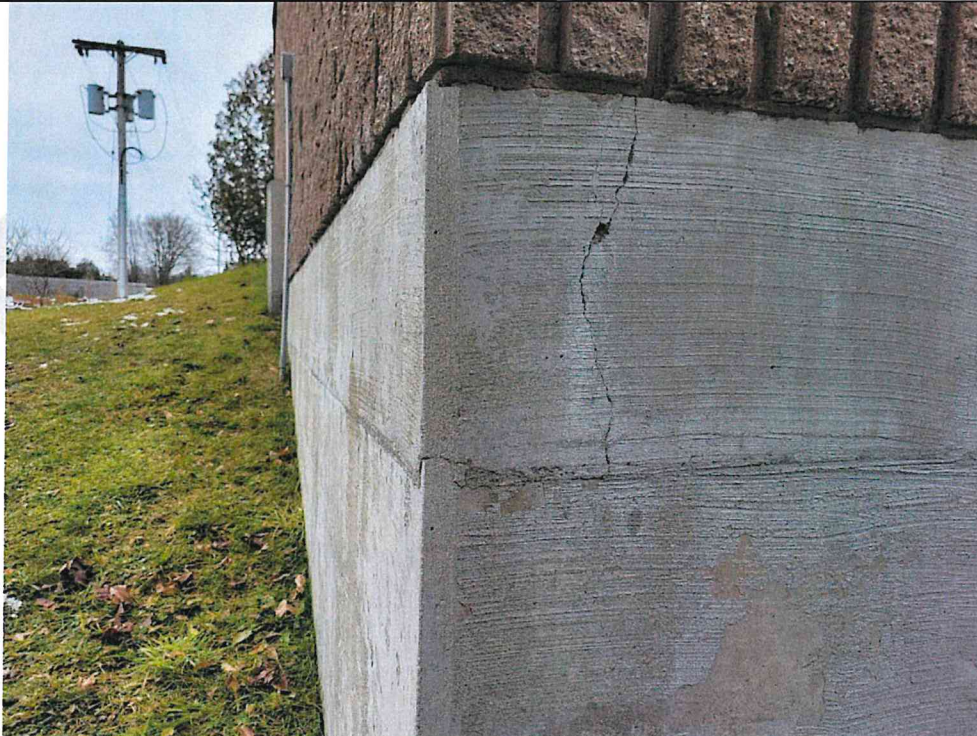
Photo S10: Suspended Slab. Cracking on Exterior SW Corner
