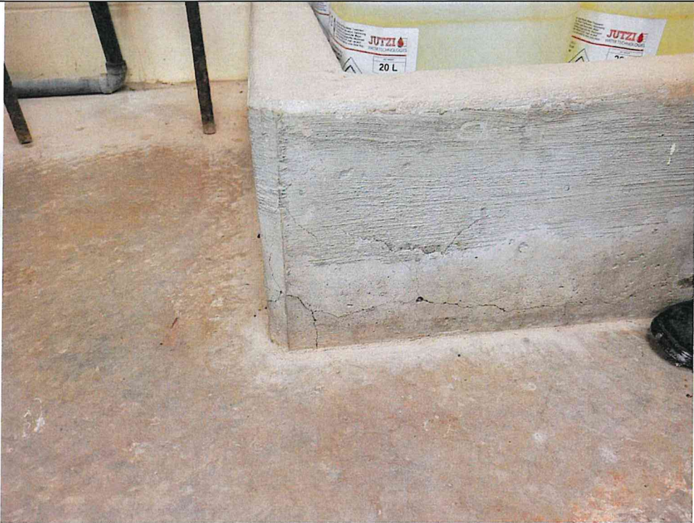
Photo S14: The Containment Curb is Cracked. Wall is Approx. 100mm Thick
