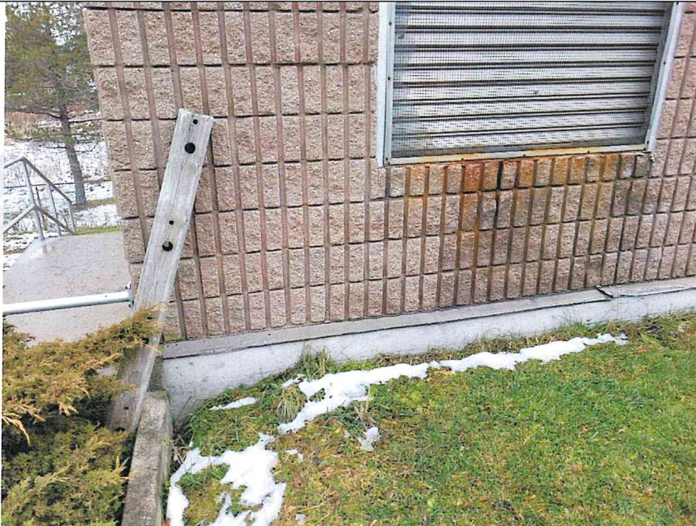
Photo S22: Block Veneer. Staining at Louver
