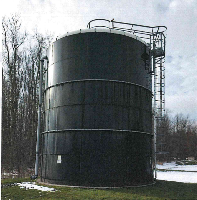
Photo PPE21: Standpipe. Sealant Dripping on the Exterior.
