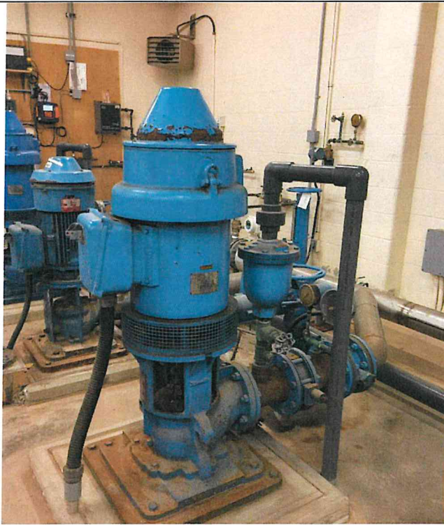
Photo PPE2: High Lift Pump #3. Pump is Not in Operation.
