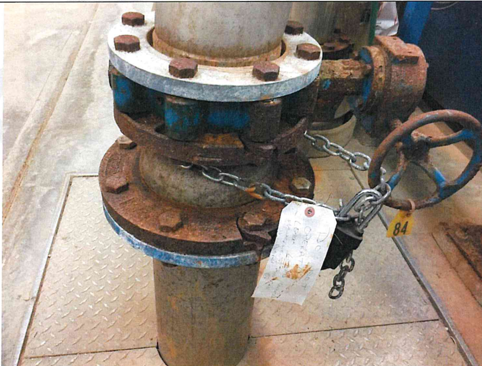
Photo PPE9: Well Pump 2 Discharge Butterfly Valve. Heavily Corroded.
