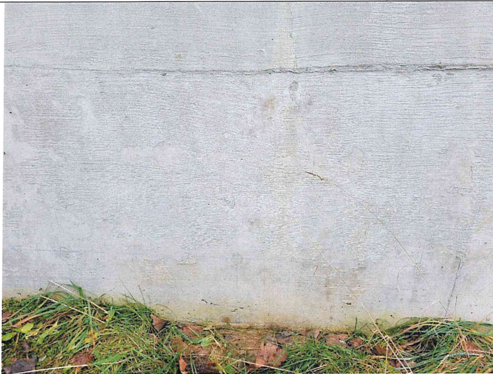
Photo S11: Strip Wall Foundation c/w Footing. Shrinkage Cracking w/ Possible Chemical Leakage
