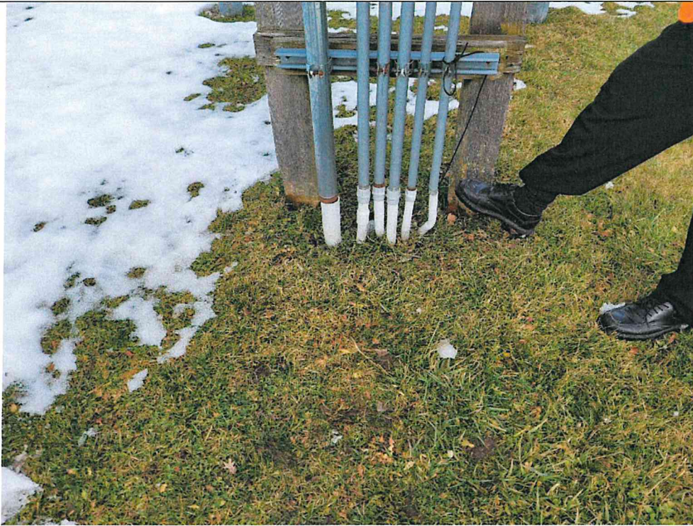
Photo S29: Electrical Panel Wood Post Support is Rotted at Base.
