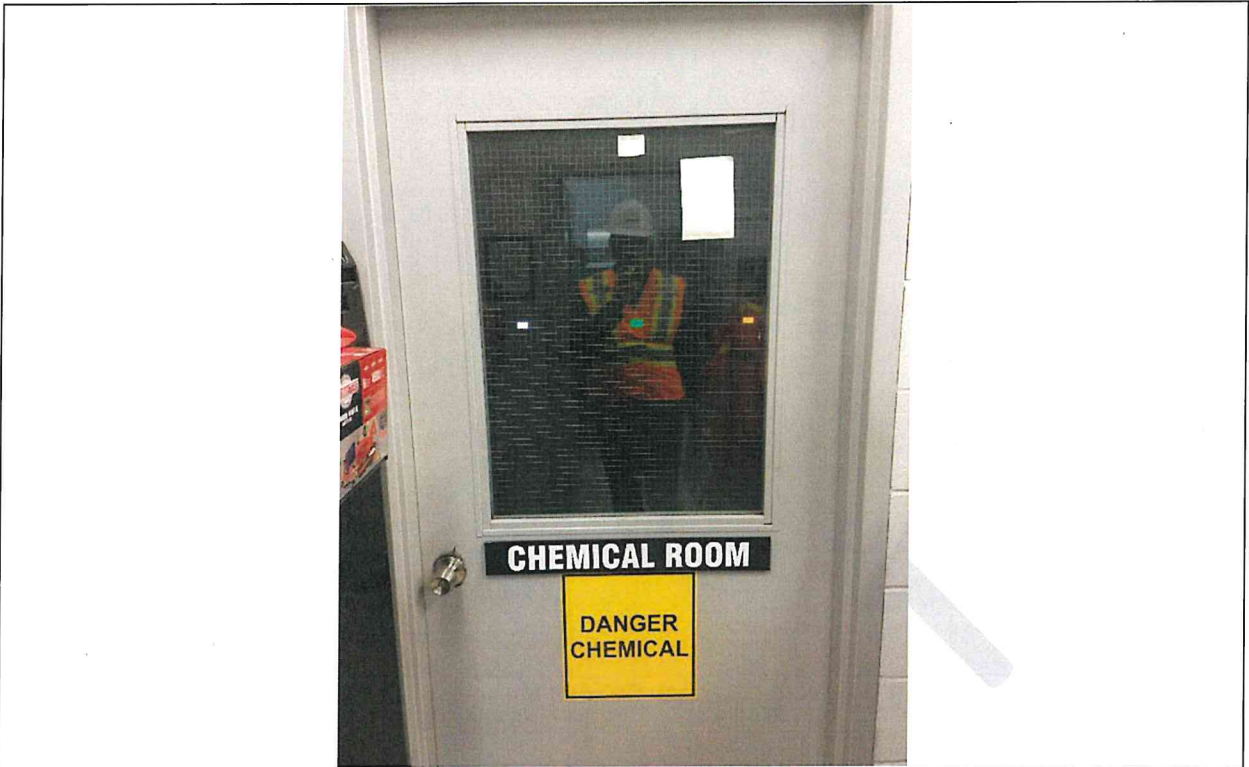
Phot BE5: Emergency Lighting. No Emergency Lighting Observed in the Chemical Room.
