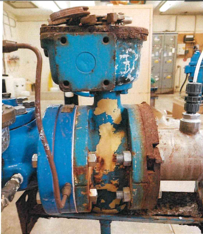
Photo PPE8: Well Pump 1 Discharge Butterfly Valve. Mild Corrosion.
