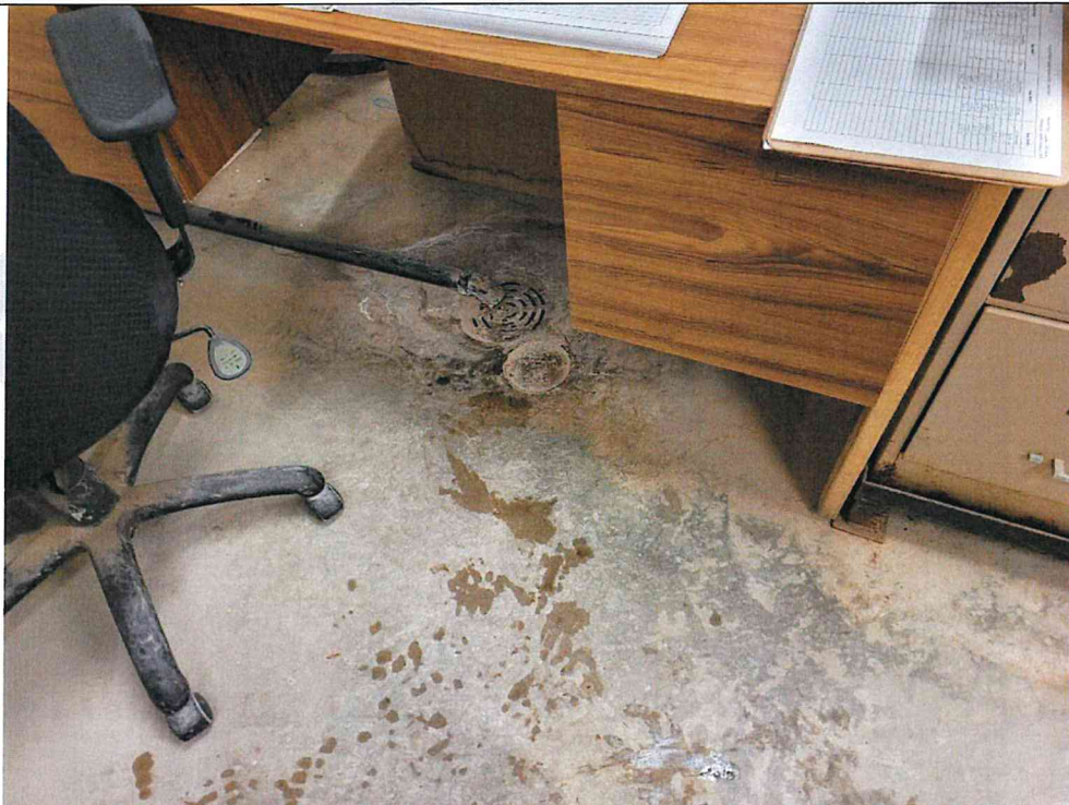
Photo S8: Suspended Slab Inside Pumphouse. Signs of Ponding
