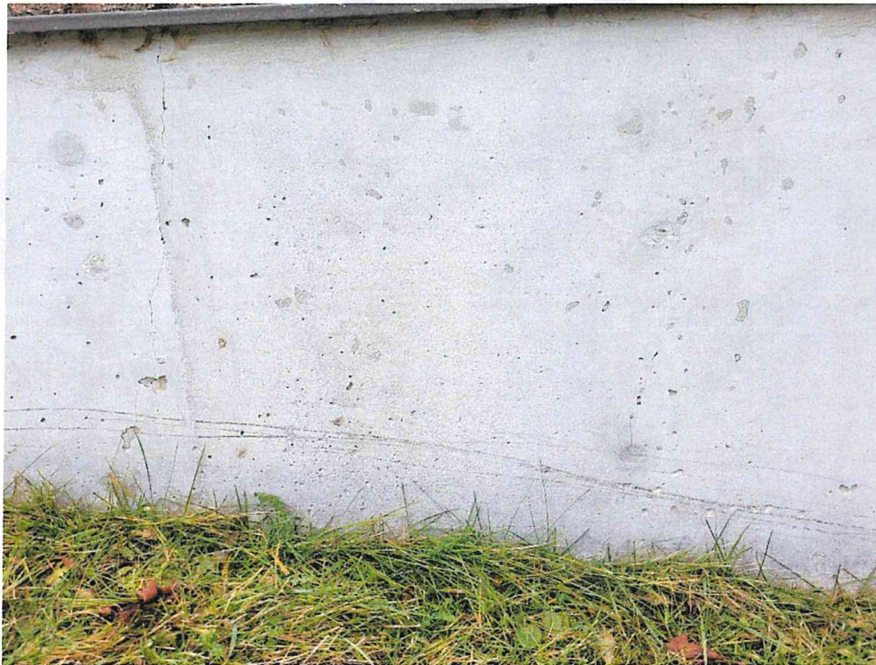
Photo S2: Reservoir Walls. Only Partially Exposed. Shrinkage Cracking on SE Corner
