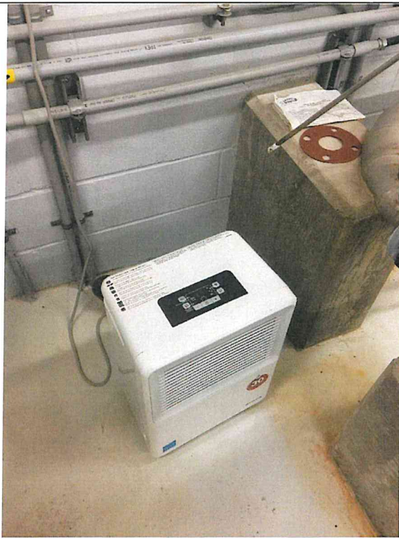
Photo M3: Portable Dehumidifier. Good Condition, but Lacks Capacity to Dehumidify Entire Space.
