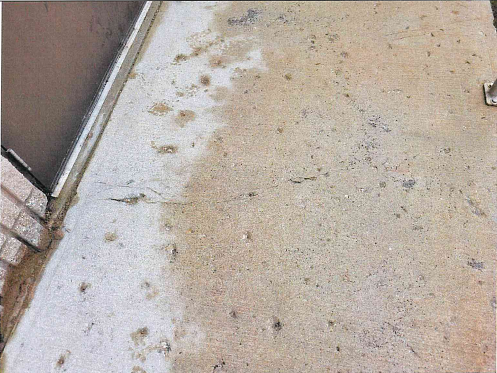
Photo S16: Concrete Stairs c/w Landing. Cracking and Localized Spalling
