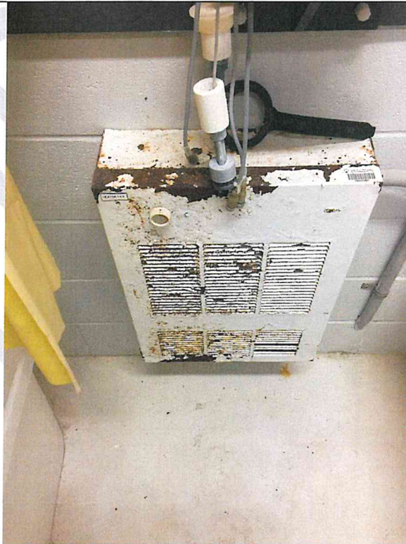
Photo M4: Unit Heater (Chemical Room). Considerable Corrosion of Enclosure.
