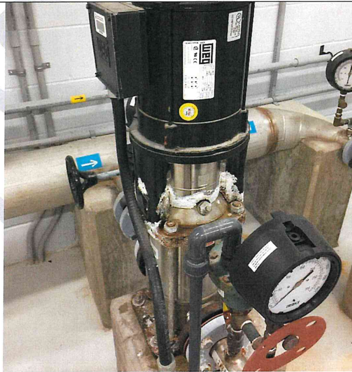
Photo PPE25: HLP #2. Corrosion and Build-up.
