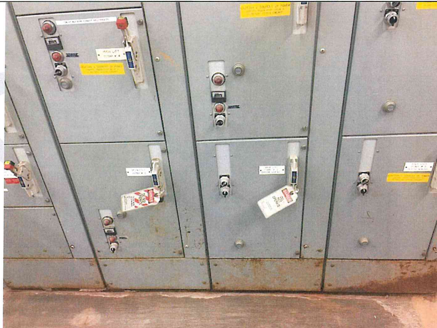
Photo PE2: MCC. Poor Condition, Limited Spare Capacity. Consider Replacement.
