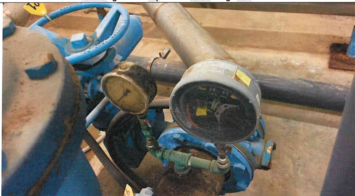
Photo PI5: High Lift Pump 05 Pressure Gauge. Poor Condition.
