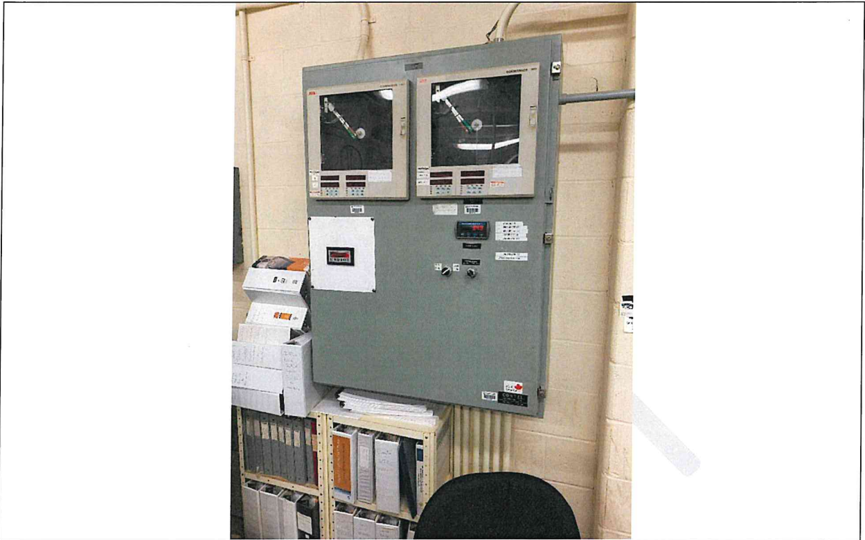
Photo PE5: Chart Recorder Panel. Fair Condition, Some Rust. Consider Merging with PLC Panel.
