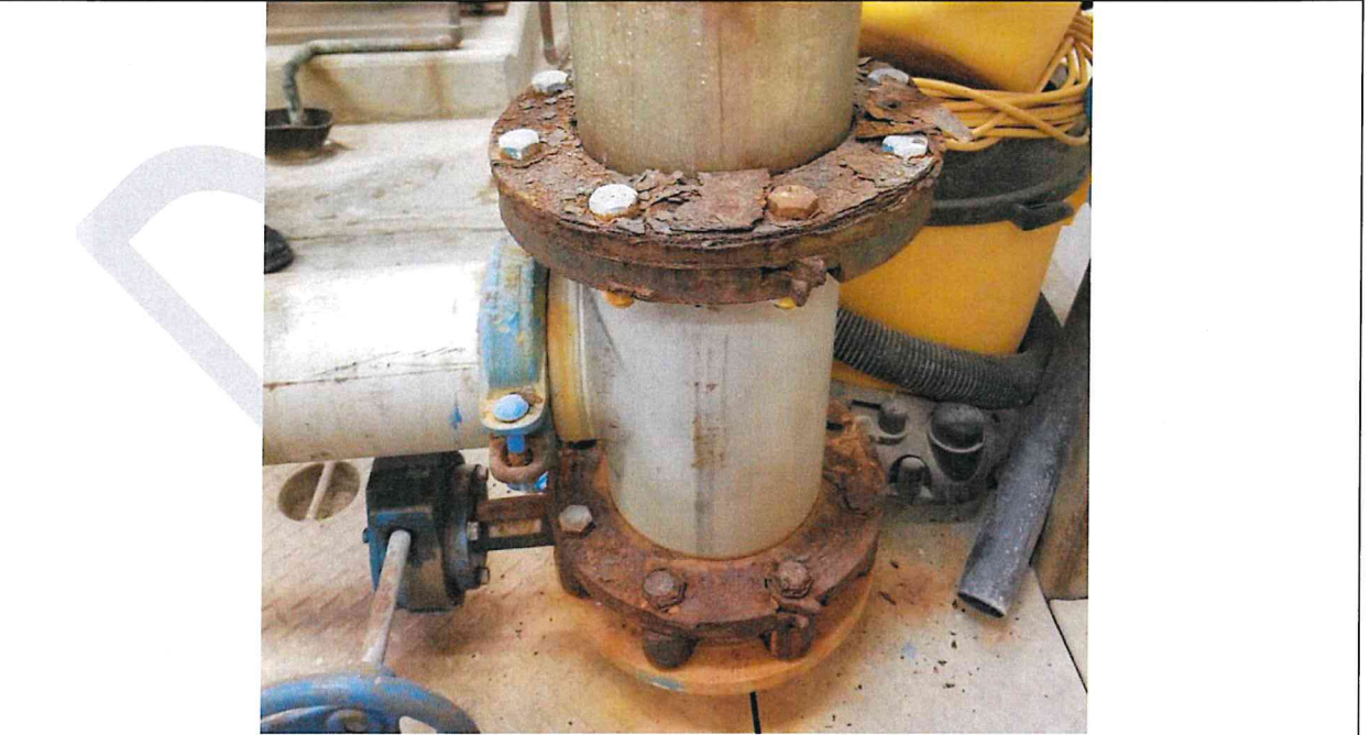
Photo PPE11: Well 2 Isolation Valve and Wells Common Discharge Valves. Heavy Corrosion.
