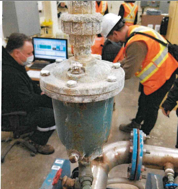
Photo PPE7: Well Pump 1 Air Release Valve. Heavily Corroded.
