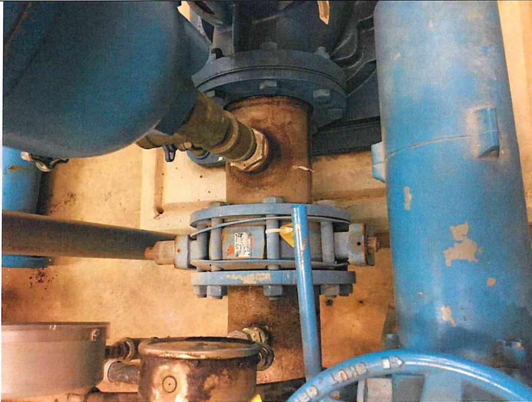
Photo PPE17: High Lift Pump 5 Pipe. Heavily Corroded.
