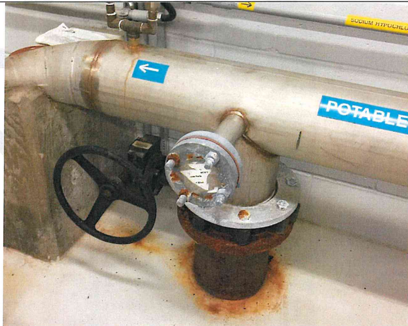
Photo PPE23: HLP1, HLP2, HLP3 & HLP4 Piping and Appurtenances and Valve Stanpipe to Suction Header. Corrosion in Water Pipe.
