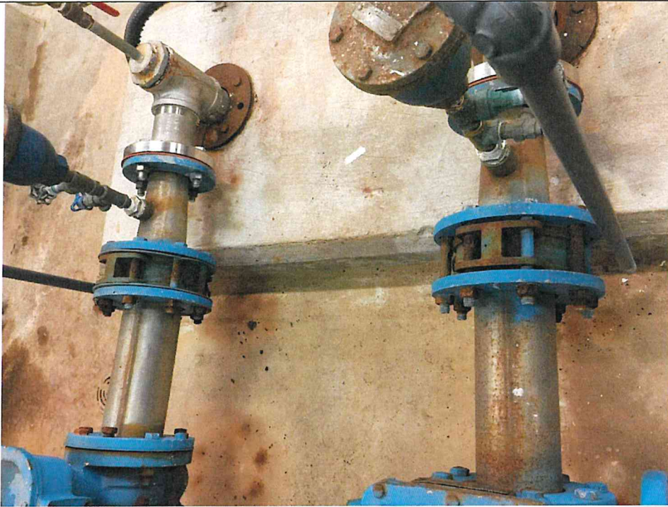
Photo PPE16: High Lift Pumps 1 and 2. Corroded Pipe.
