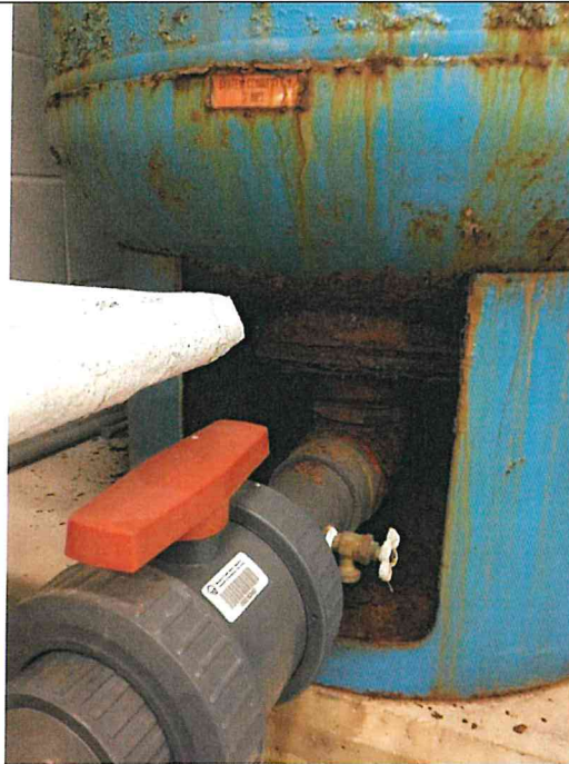
Photo PPE26: Pressure Tanks. Heavy Corrosion.
