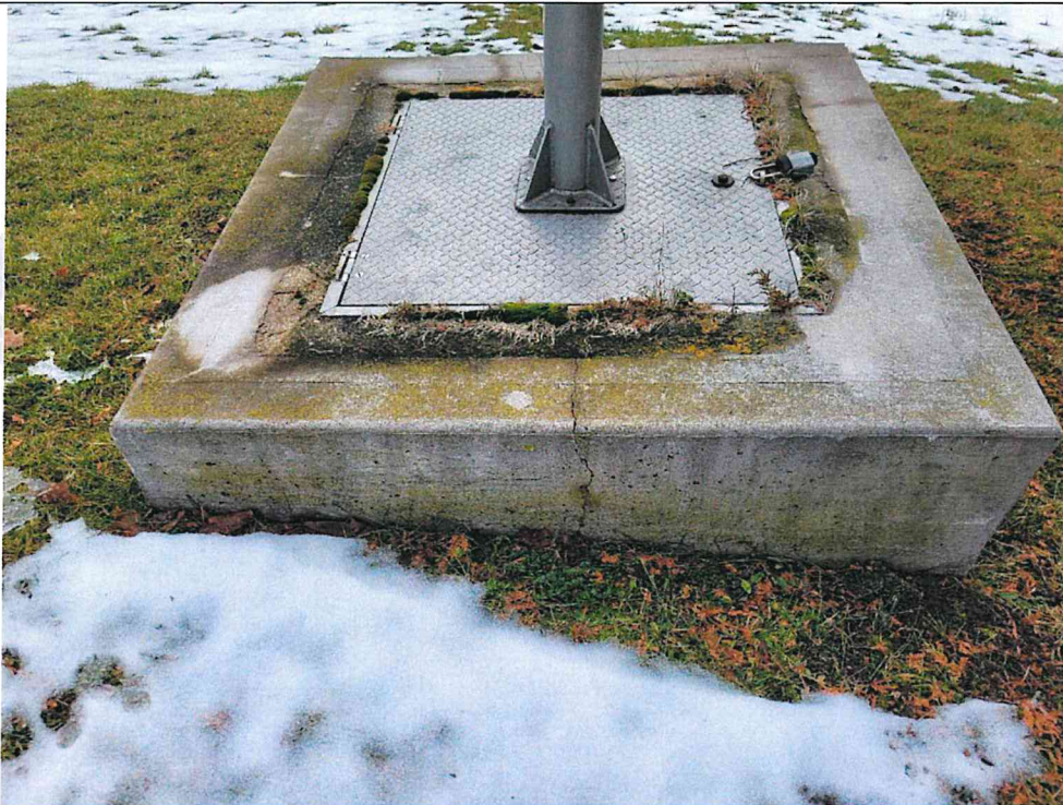
Photo S6: Reservoir Access Chimney. Vegetation Growing on the Concrete Collar. Collar has Vertical Crack.
