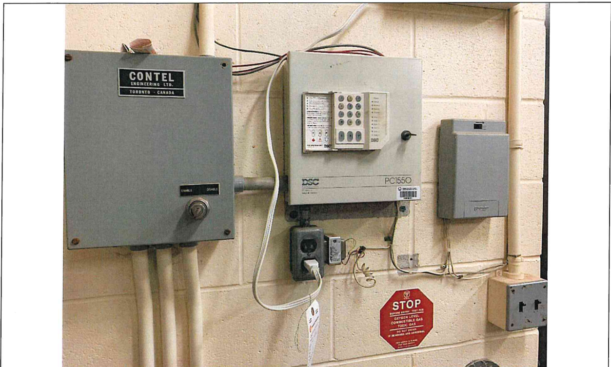
Photo BE1: Building Alarm System (Including Autodialler) Lacks Bandwidth for Additional Alarms.
