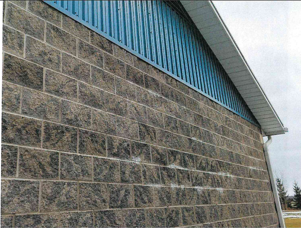
Photo S37: Staining on Block Veneer.
