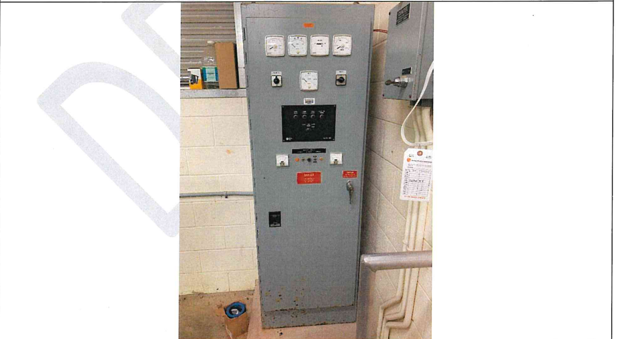
Photo PE4: Battery Charger Panel. Poor Condition. To be Removed upon Genset Replacement.
