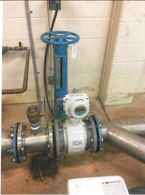
Photo BE3: Building Conduits & Receptacles. Some Conduits in Poor Condition. Flowmeter (pictured) Does Not Use Conduit to Carry Signal Cable to PLC Panel.
