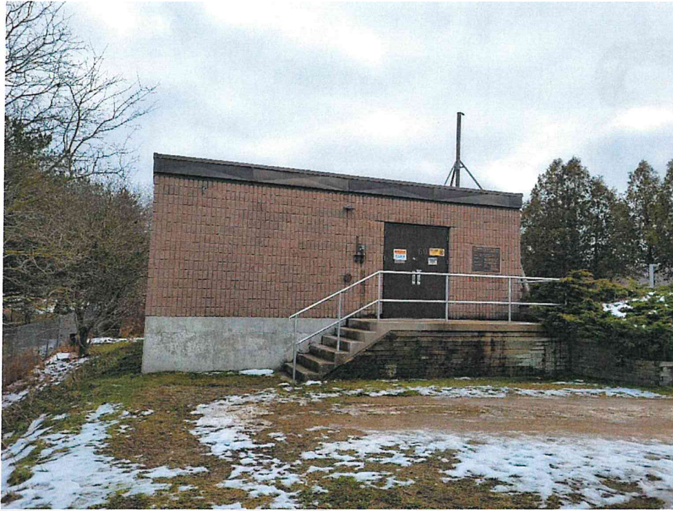
Photo S1: Drayton Pumphouse and Reservoir
