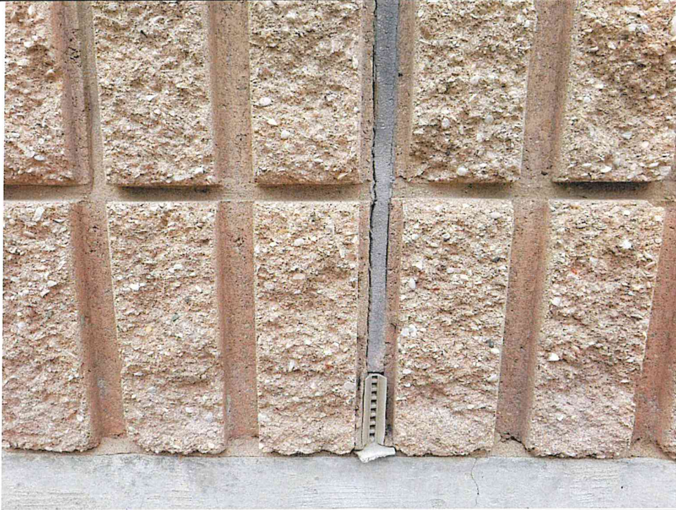
Photo S23: Block Veneer. Failed Sealant
