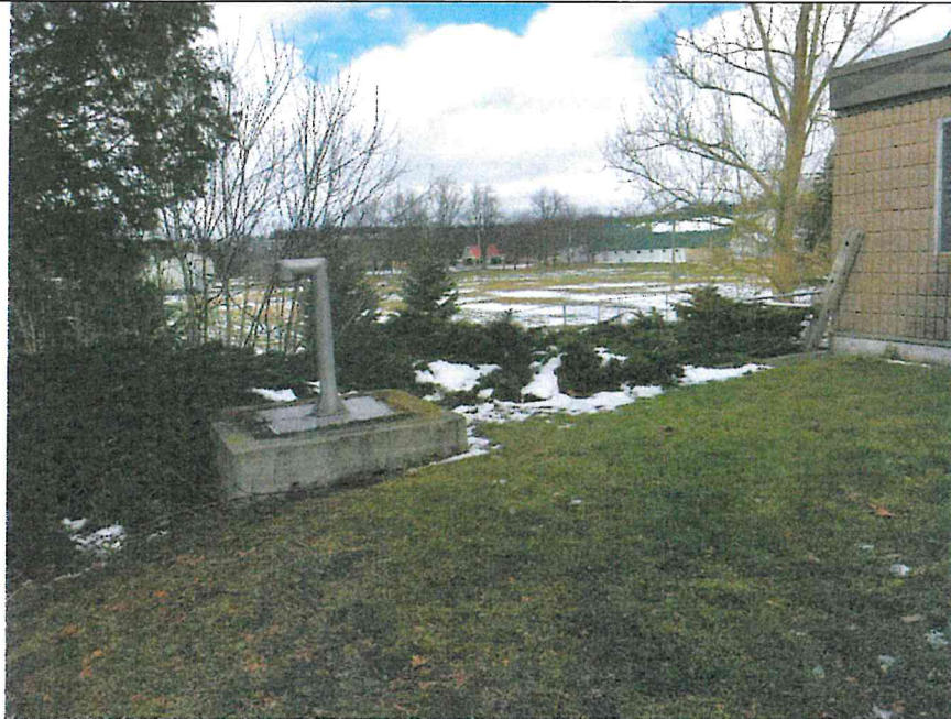
Photo SW2: Trees and Bushes. Reservoir Hatch Drains are Clogging.
