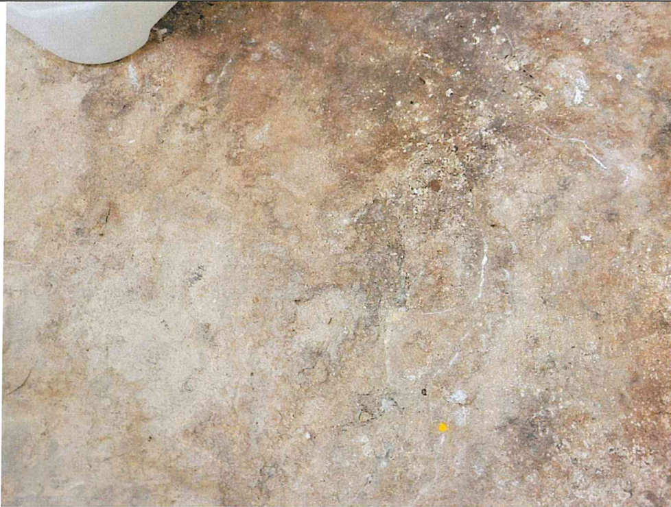
Photo S9: Suspended Slab Inside Pumphouse. Chemical Damage at Containment Areas
