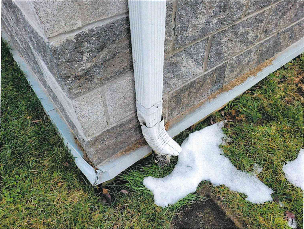
Photo S38: Bend Downspout. The Splash Pad is Too Far From the Downspout Lead.
