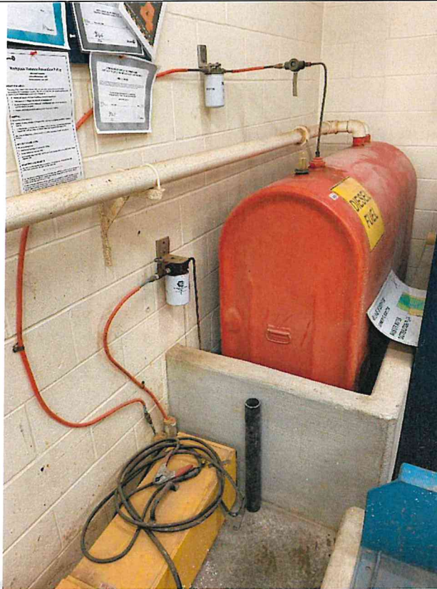
Photo M1: Genset Fuel Tank. To be Removed Upon Replacement of Genset.
