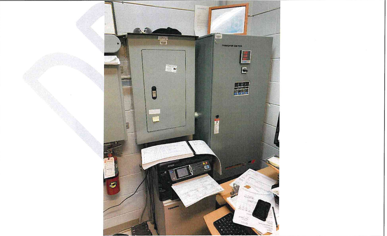
Photo BE6: Automatic Transfer Switch. Improper Storage of Desk within Unsafe Proximity of Electrical Equipment.
