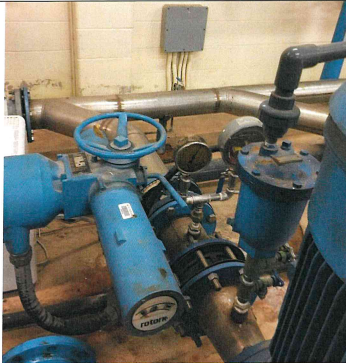
Photo PPE20: Piping and Minor Appurtenances HLP 5. No Flowmeter.
