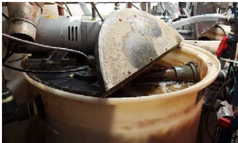
MBBR Pilot Testing Equipment
