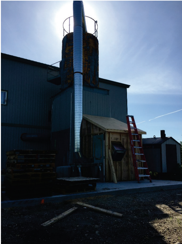
Figure 1 – Dust Collector 1 with Silencer and Enclosure Installed.
